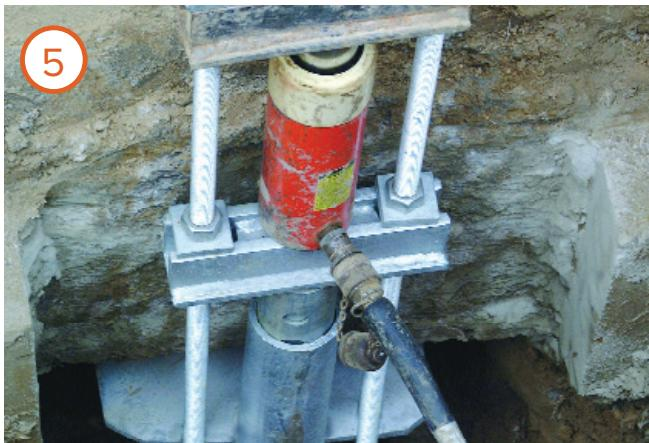
The foundation wall may be lifted to the desired elevation and the structure is permanently stabilized.
