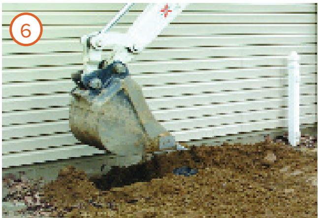
Cracks below the surface level of the landscape are repaired, the excavation is back-filled, and the project is completed.
