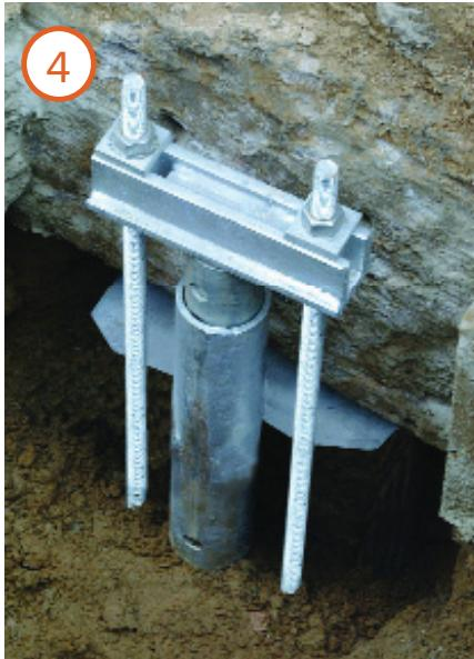
Once the piles are drilled to the required depth, the bracket is installed and the weight of the wall is transferred to the helical pile assembly.
