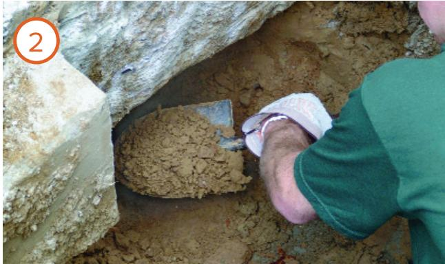
Next, we notch the footing and prepare for placement of the patented IDEAL underpinning bracket.
