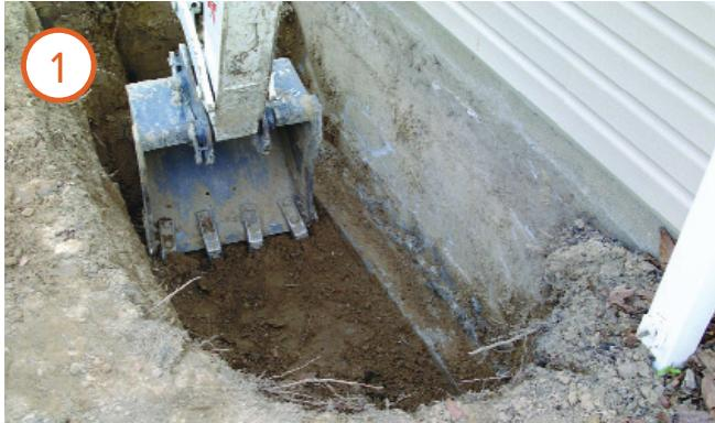
First, we excavate down to the footing of the affected foundation wall.
